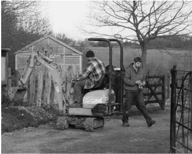
Working on the new water supply.
