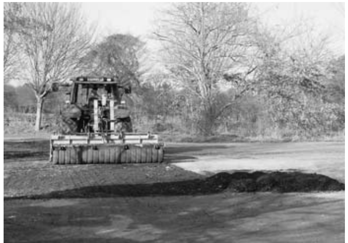
Agripower resurfacing the car park in February
