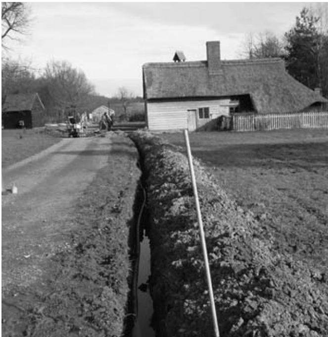
The trench runs smoothly, anyway . . .
