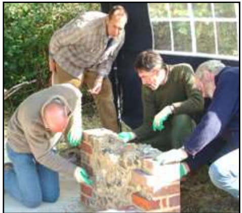
Chilterns Vernacular Building Skills Course working with Lime, flint and brick
