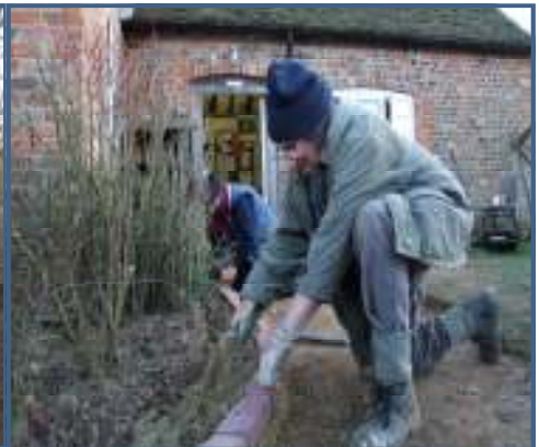
Site volunteers building the new brick path to the Volunteers room
