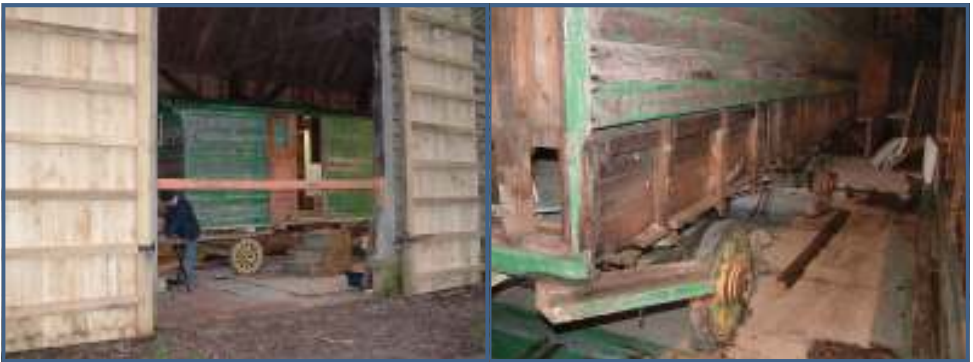
Repairs on the Living Van in Northolt Barn
