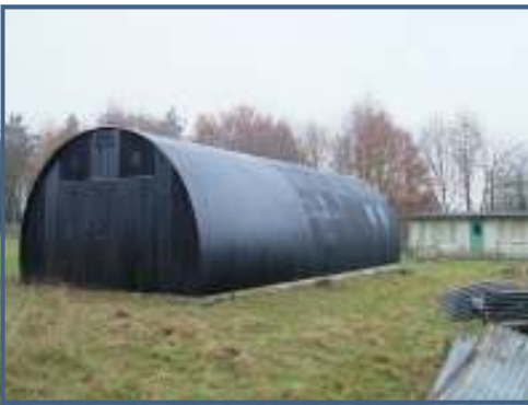
Nissen Hut from Sewell now completed
