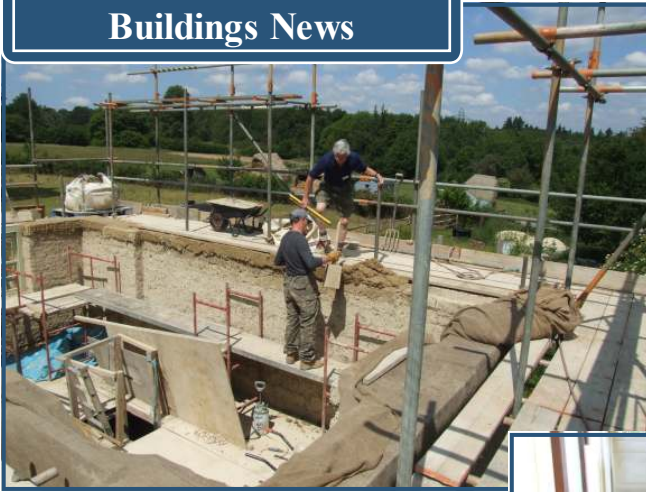
Above - Work restarts on Haddenham Cottage
