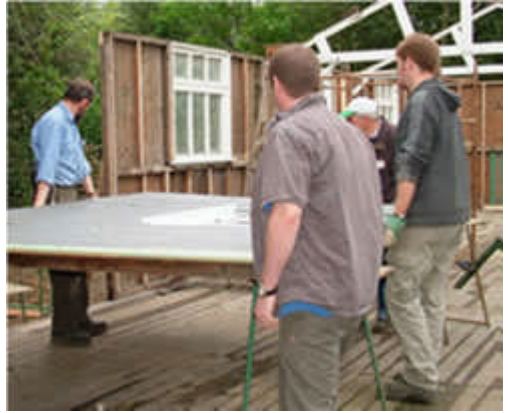
Erecting the Gerrards Cross Hut.
