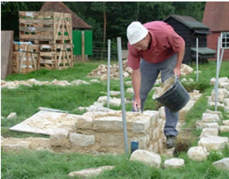
Tim Amsden laying grumplings.
