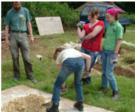
Mixing mortar for grumplings.
