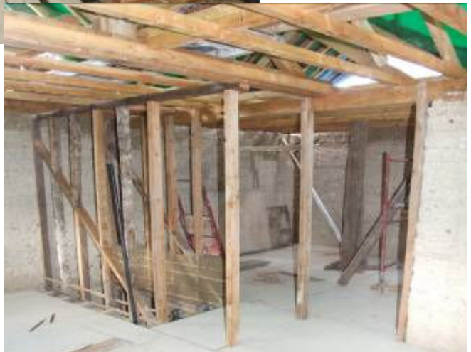
Internal wall on the first floor of Haddenham Croft Cottage
