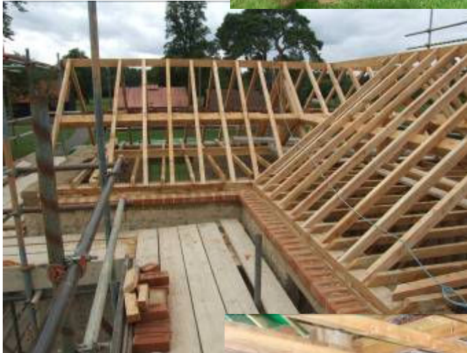
Haddenham Croft Cottage roof under construction
