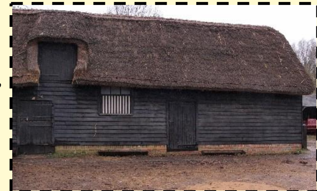
Marsworth Cattle Shelter, Stable & Cart Shed clad in weatherboard
