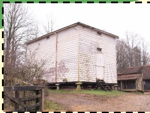
Rossway Granary clad in weatherboard
